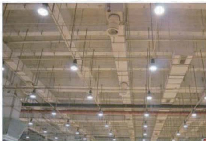
Commercial application: Exhibition Room, Gas Station, Supermarket etc.
